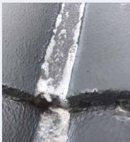
Cleaning your roof helps remove the environmental fallout.
